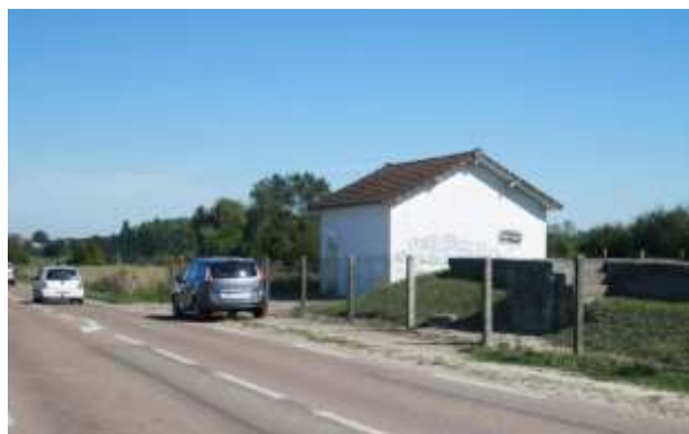
Station de pompage
